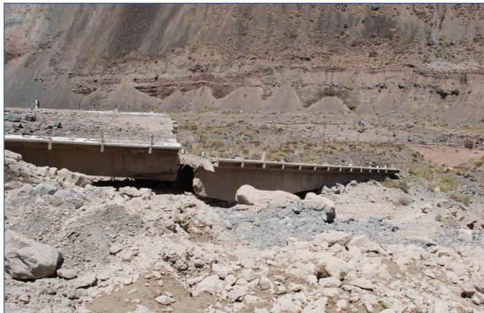
Fig.67: There could hardly be a greater demonstration of the ferocious power of the storms than this: the road broken and swept to one side by a rock avalanche. (15 Jan 2013. JMW)
