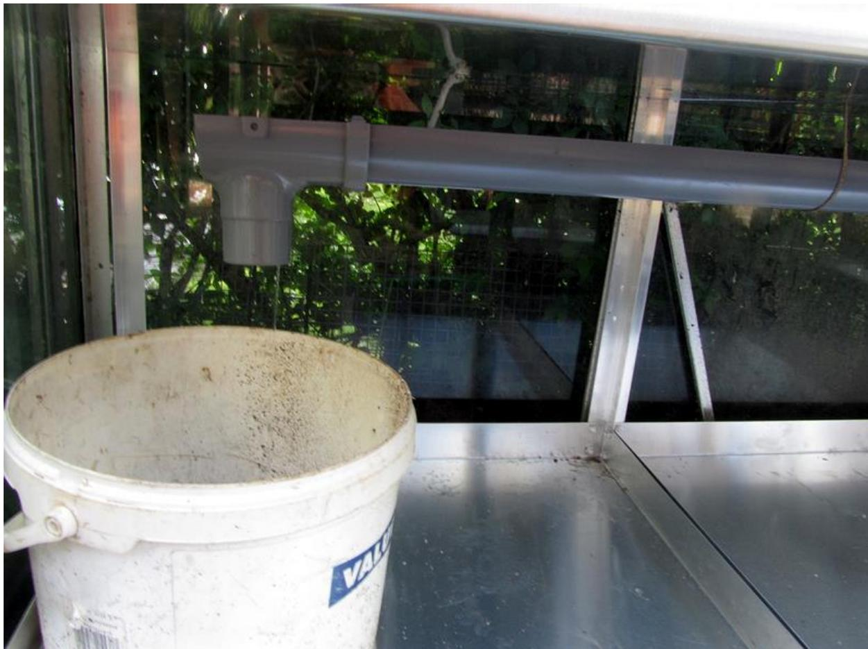
A bucket or watering can will be placed there to catch and recycle the water that drains away.
