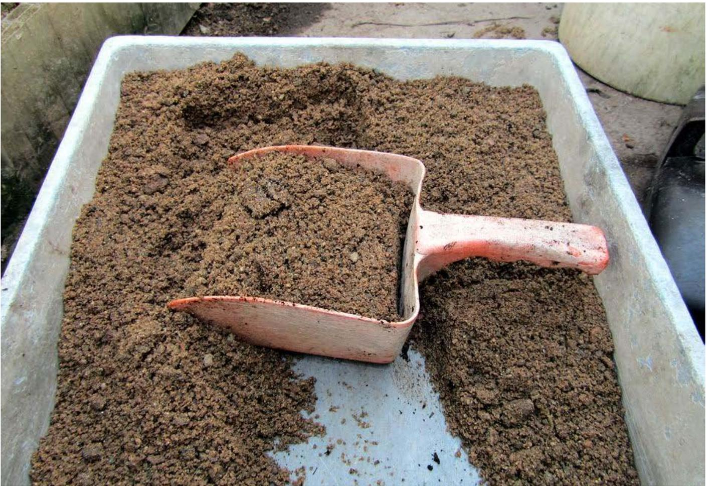
I measure the quantities for the mix by volume using in this case a plastic scoop but for the bigger quantities I mix in the cement mixer I would use a bucket.
