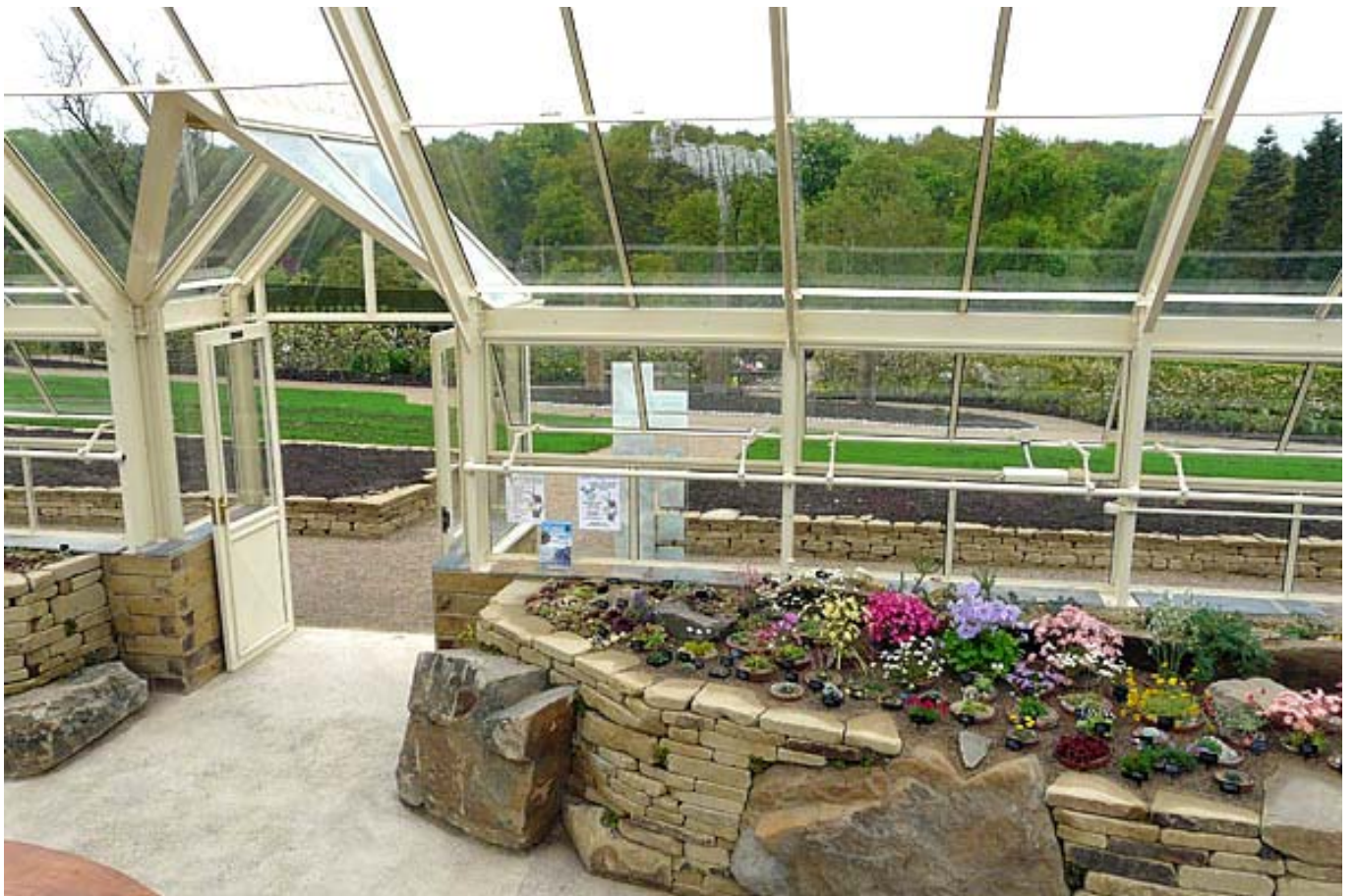
The new glasshouse is well ventilated with ridge vents along the whole top of the glasshouse,
