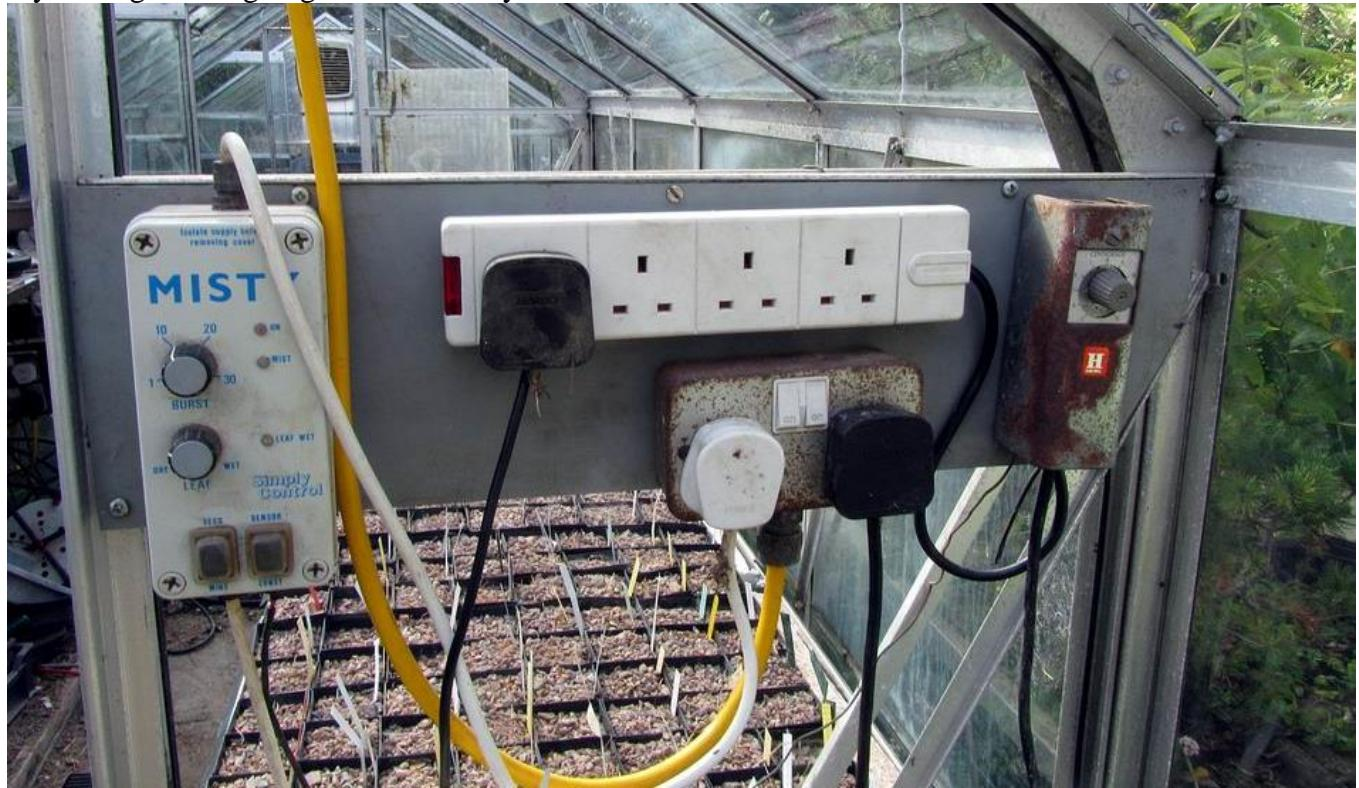
I rewired the electrics giving me the mist unit control, a two outlet mains socket and a four outlet bar wired through the thermostat on the far right to control all the heating cables in the plunges old and new. All my outside electrics are protected by a leakage to earth trip switch
