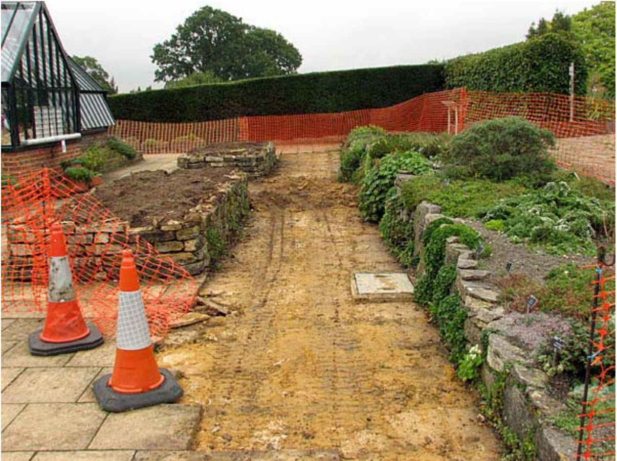
It had taken about 3 working days to get to this stage. Peter and Chris moved on to demolishing the two empty raised beds, while Chloe, Lucie and Anita rescued plants from the remaining bed.
